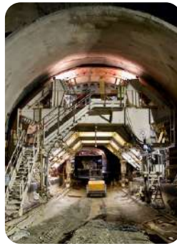
Tunnels and major public works
