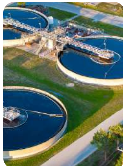
Waste treatment plants
