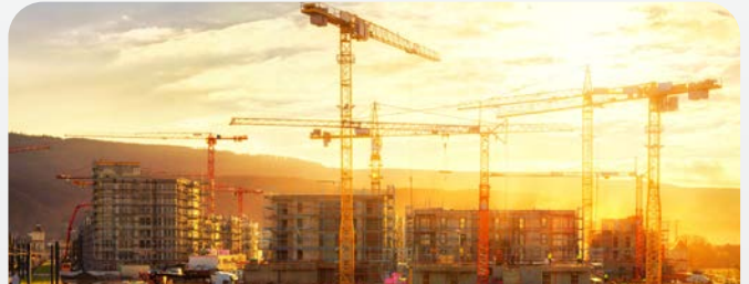
CONSTRUCTION, REMEDIATION, DEMOLITION
